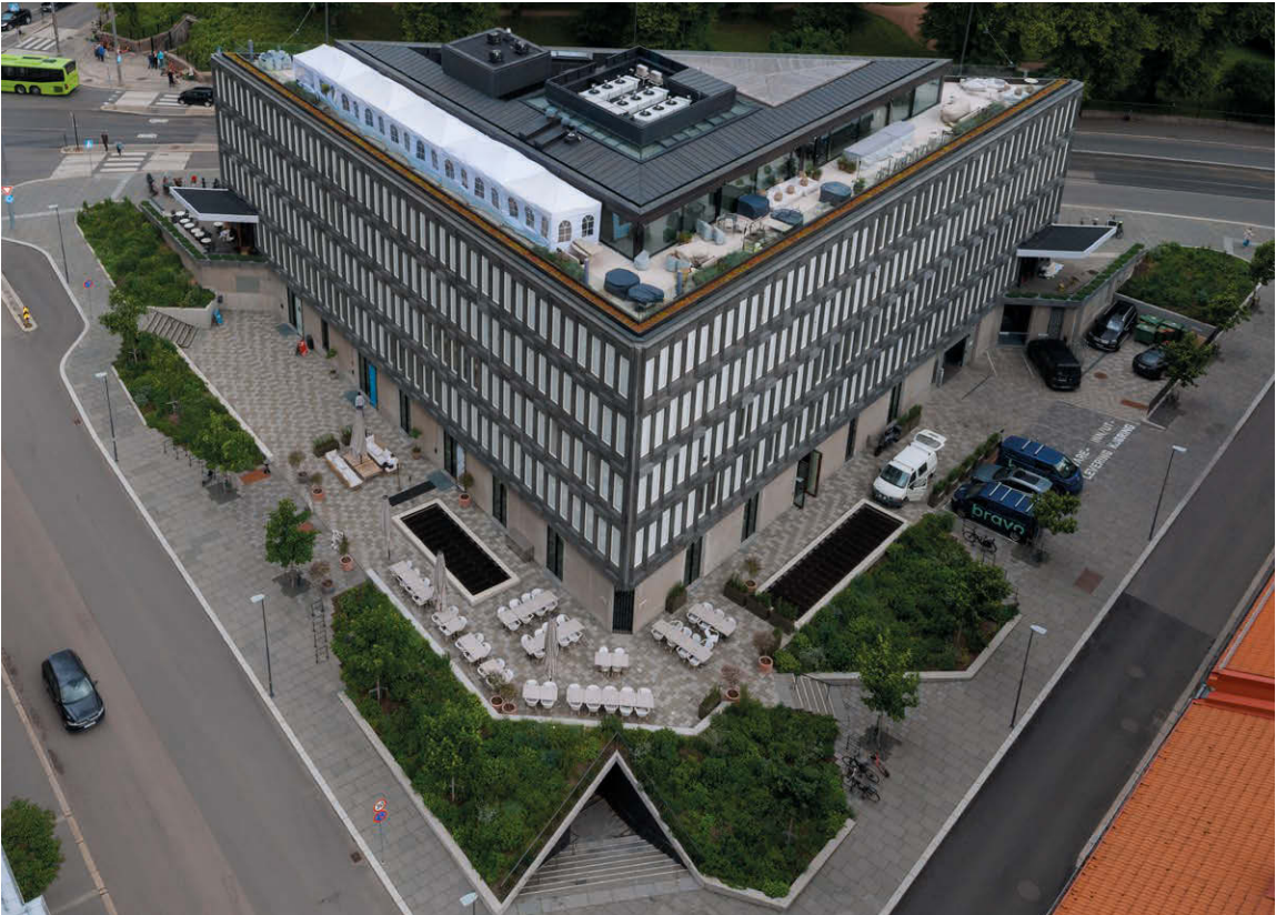
By relocating the extensive building services to the basement, the top floor became freely accessible for a restaurant and roof terraces.
